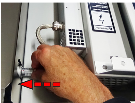
26. Reconnect the power wire.
