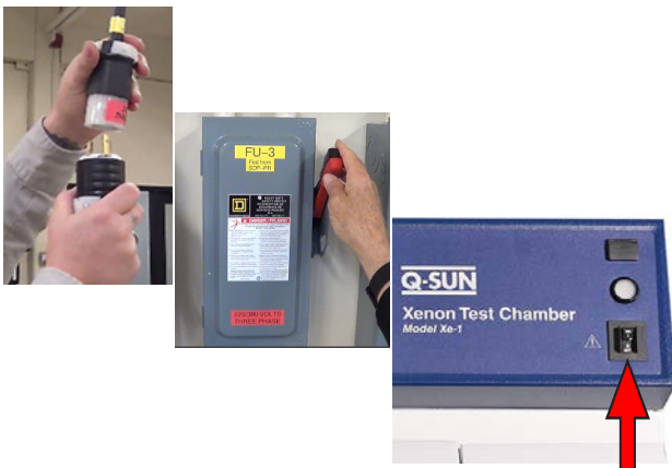
28. Reconnect Power. Power ON . Xe-1 power ON .
