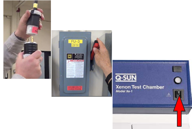
22. Reconnect Power. Power ON. Xe-1 power ON.
